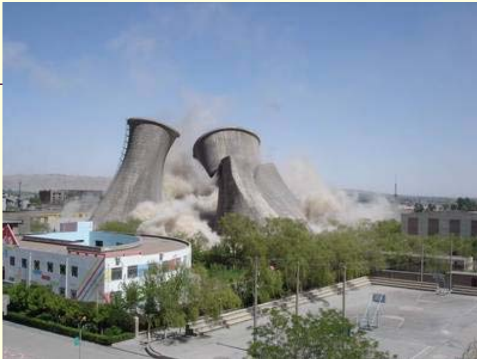
The first blast for energy saving in Gansu Province. No.1-No.3 cooling towers of Yongchang fire power station were exploded after operated 40 years.
