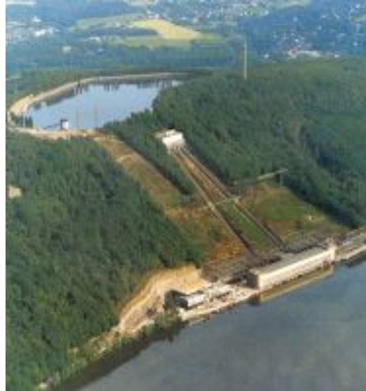
Herdecke pumped storage plant Germany
